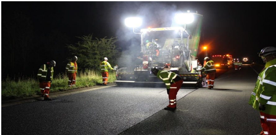
Laying (off paver)
